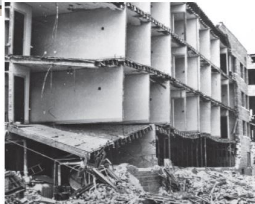
1925 Santa Barbara, California Earthquake Unreinforced Masonry Damage to the Hotel California
