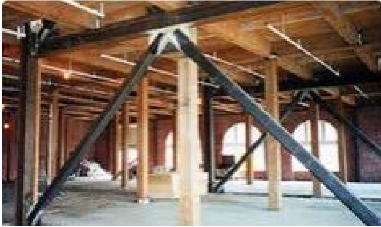
Interior cross bracing helps prevent building collapse
